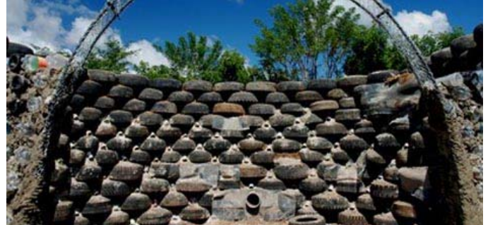
Figure 11: Car tires for an earthship wall
