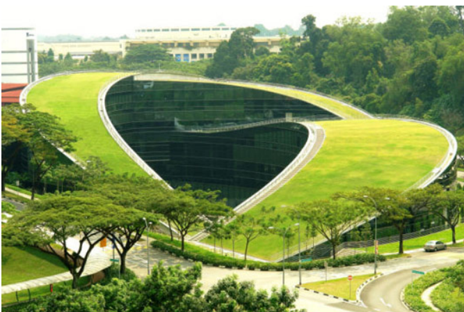
Figure 5: A spectacular green roof
