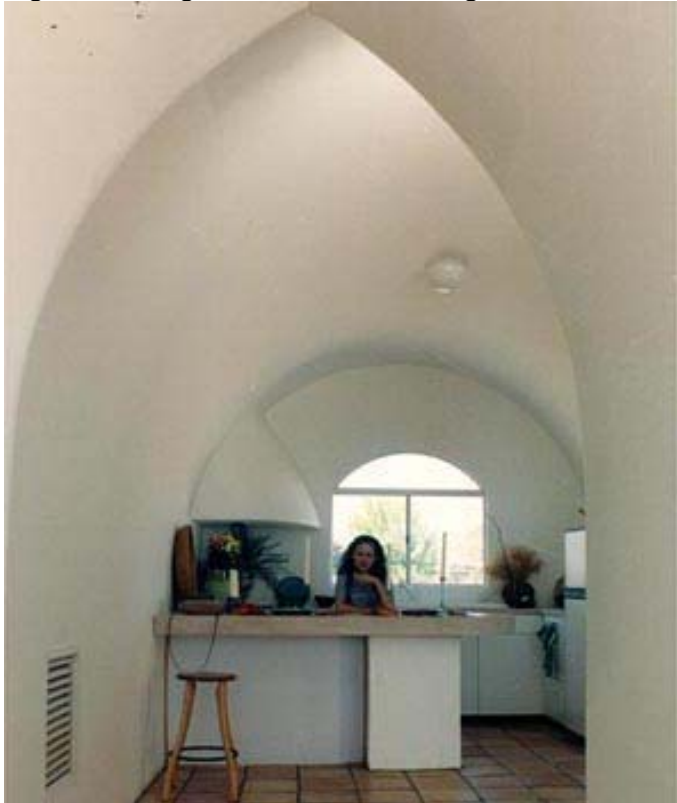
Figure 10: Interior finishing of an earth bag house
