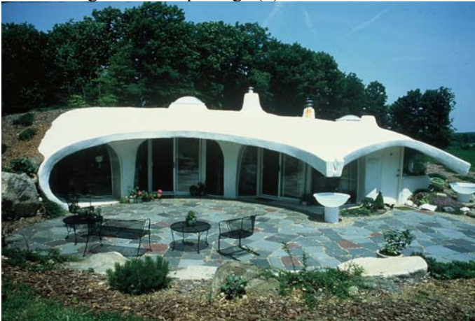
Figure 4: A partial earth shelter
