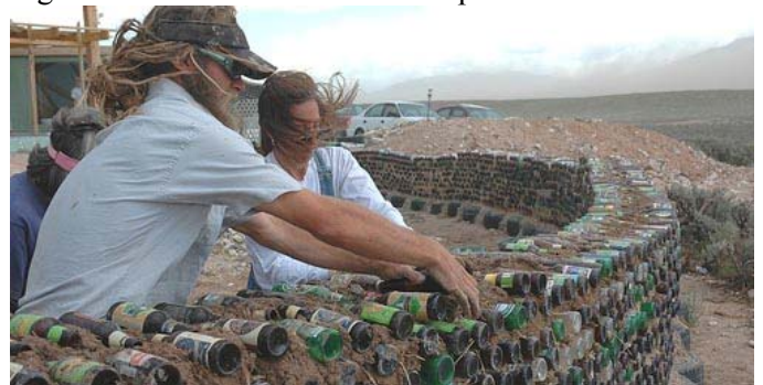
Figure 12: Bottles for an earthship wall
