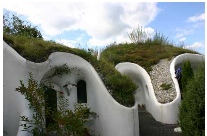
Figure 3: The use of concrete for ESB
