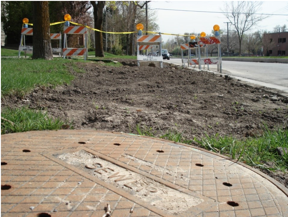
Figure 2: Surface location after installation of the exterior heat exchanger system
