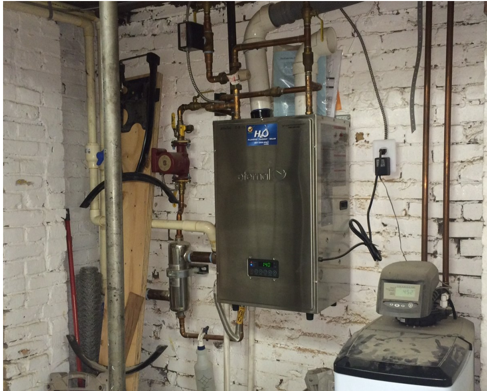
Figure 6: Tankless gas water heater
