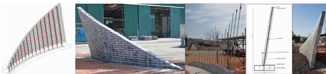
Figure 1 Axonometric view, steps of building and section of the stone sail with revealed the system of reinforcements.
