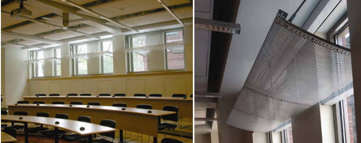
Figure 4: Light shelves and ceiling fans in a south-facing Lillis classroom (left photo courtesy of Emily J. Wright; right photo courtesy of SRG Partnership).
