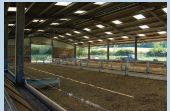
Open-sided sheds allow good airflow in sheltered locations. Yorkshire boarding or webbing may be needed in more exposed sites
