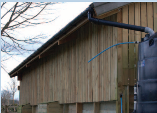
Yorkshire boarding can be used to allow good ventilation while blocking driving rain in exposed sites
