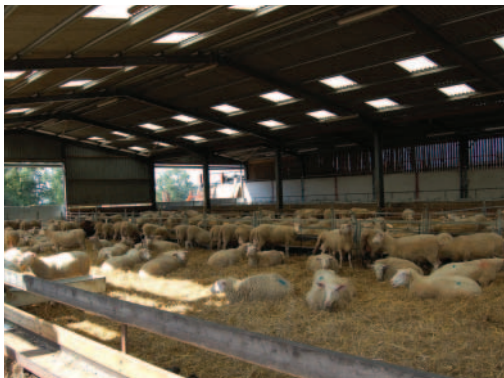
Well-ventilated housing is essential for reducing levels of respiratory disease in sheep. This shed has an open central ridge, a low stocking rate, an open sheltered side and Yorkshire boarding on the more exposed side; there are also air inlets at either end, allowing good airflow throughout
