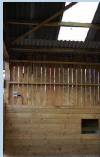
(right) The solid lower wall prevents draughts at animal level, with Yorkshire boarding above to provide a fresh air inlet. (below) An open ridge enables the warm, stale air to escape and allows the circulation of fresh air in ridged buildings
