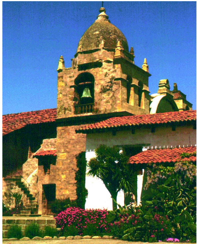
Figure 1: Historic buildings often come with a variety of useful elements that can be reused or can help lower the heating and cooling loads on a new HVAC system. In this California mission, heavy adobe walls, deep tile roof overhangs, covered verandas, the bell tower and the high interior nave, all work to reduce the heat build-up and move air through the building. Architects and engineers should include these passive benefits when calculating energy loads.
