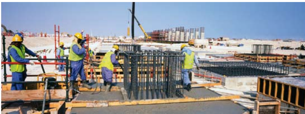
Pearl GTL construction
