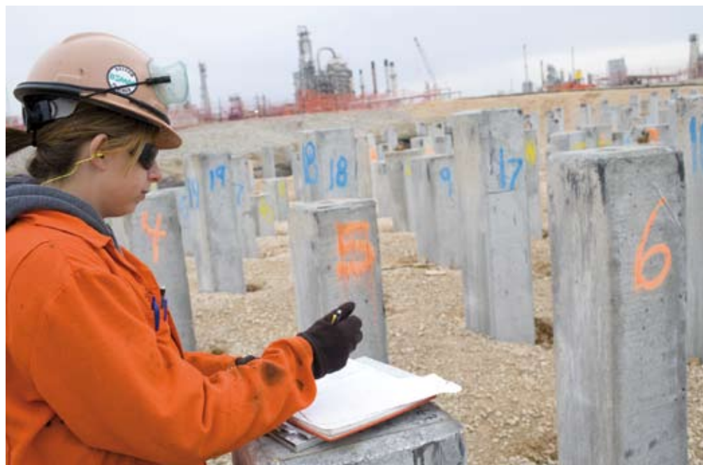
Construction at Port Arthur
