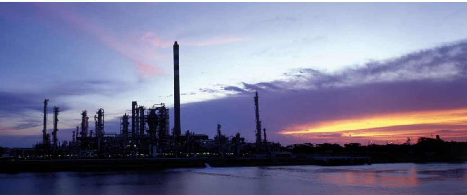
The Long Residue Catalytic Cracking Unit (LRCCU) on Pulau Bukom
