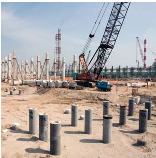
Construction at Bukom Island
