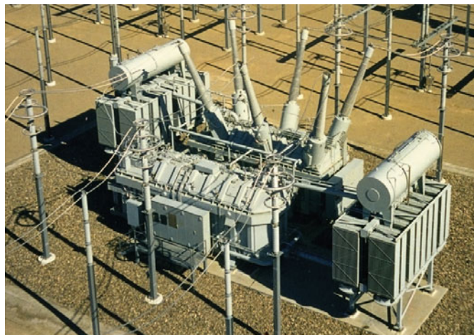
Fig. 5.7-1: Phase-shifting transformer
