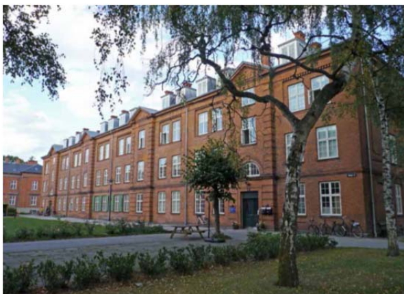
Fig. 8. Elmehuset building after refurbishment
