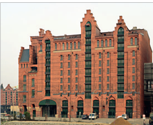
Fig. 9. Historic building reconstruction in Hamburg
