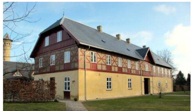
Fig. 5. Kavalergården building after refurbishment
